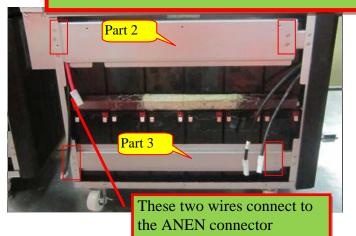
3. Screw up the Part2 & Part3 on the case by using 8 flat head screws;
